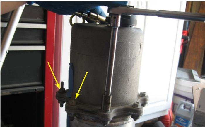
20. Using a 13 mm socket and extension, remove the eight (8) nuts and bolts on the tank to separate the top and bottom of the tank. You will need a deep well socket or an open end wrench to remove the two bolts (in which the tape is in between) indicated to the left.
