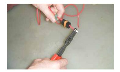
16. Using a crimping tool, crimp one of the supplied terminals onto the wire and pull the terminal back into the connector to seat it into place.
