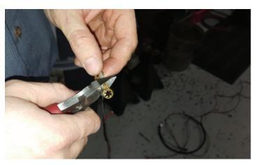
35. Cut the ring terminals off of the control wires (gray and black). Also cut off the single pin connector from the red wire. Seal up the end of only the red wire using a piece of heat shrink.
