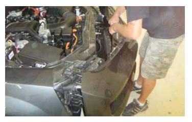
11. Remove the front fascia by gently lifting up on the top of the fascia and pulling it away from the vehicle.
